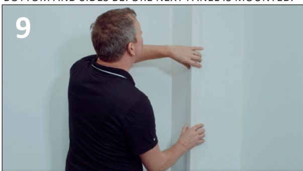
THE WALL CAN BE FITTED WITHOUT INTERNAL CORNER TRIM. FOR EXTERNAL CORNERS, OUR FLEXILIST CAN BE USED.
